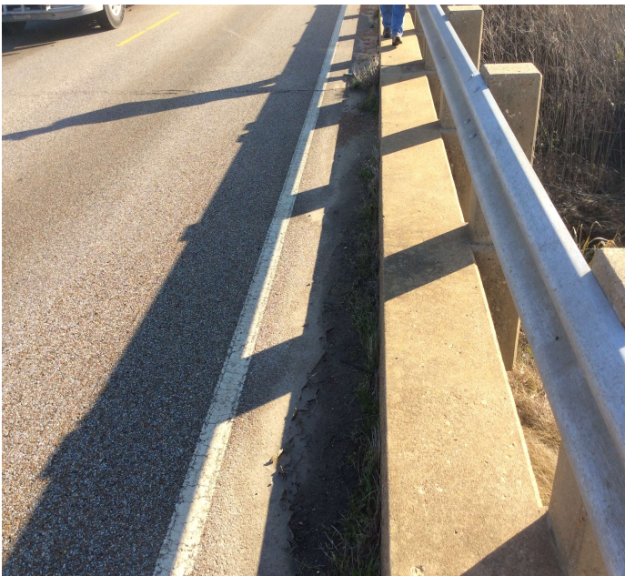
PHOTO 1 Description Vegetation is growing in gutters.
