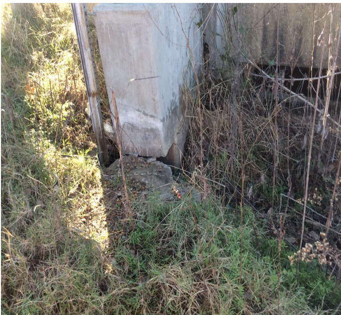
PHOTO 1 Description Abutment 2 left monument post erosion.
